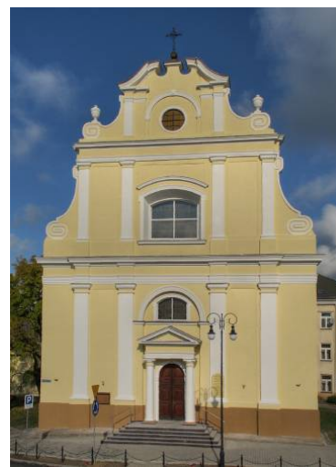
St, Trinity Church – the current view
